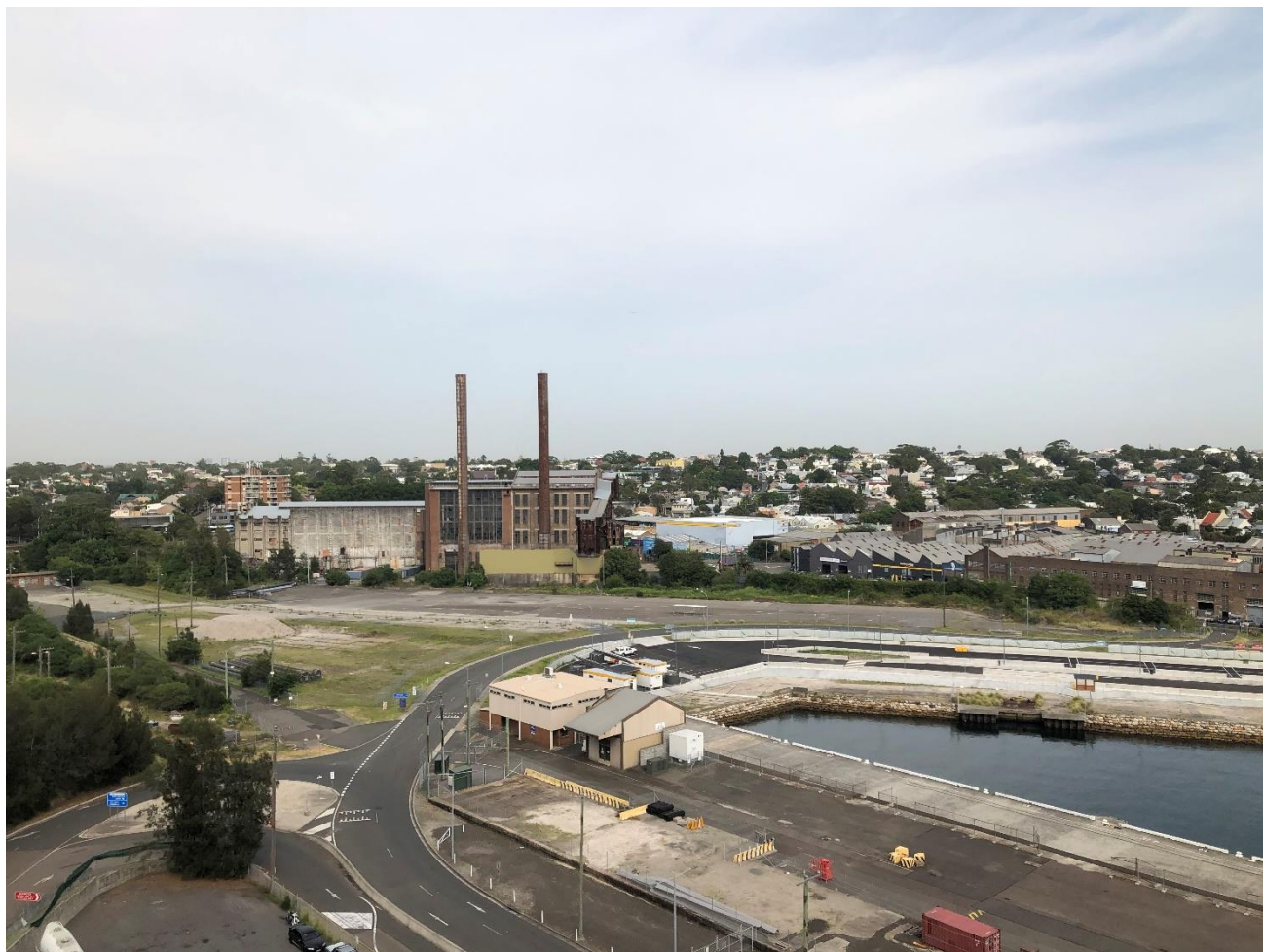
Figure 7 White Bay Power Station to the west of the site, facing west
