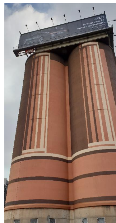
Figure 4 Glebe Island Silos, looking north-east
