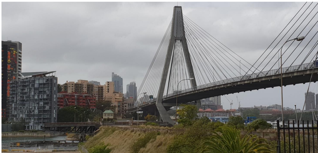
Figure 6 ANZAC Bridge, with the state heritage listed Glebe Island Bridge in the foreground
